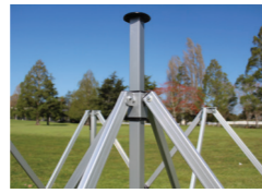
Extender peak poles with additional plastic supports to remove rubbing on roof
