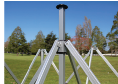
Extender peak poles with additional plastic supports to remove rubbing on roof
